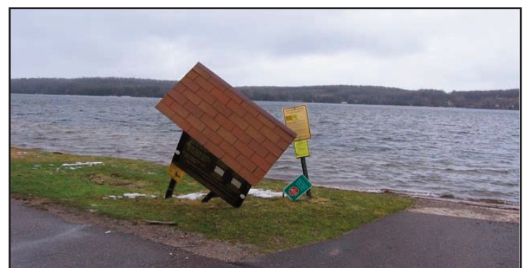
This damaged sign was removed by the Town of Phelps for safety reasons. Mike Hoffman rebuilt the one there now.
